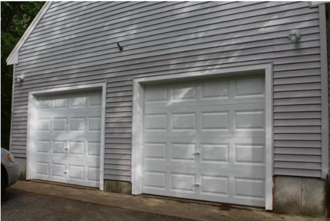
The old doors had to be replaced because their lower sections had rotted and the hardware was very rusted. While replacing the doors, we found that all the wood trim was rotted as was some of the framing. Along with those repairs, we also replaced the vinyl siding on the lower half of the garage door wall. The outside lights were also replaced in the process.
